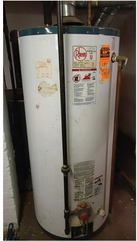
FIGURE 1-9 Schematic of an electric hot-water heater and photo of a gas hot-water heater.
